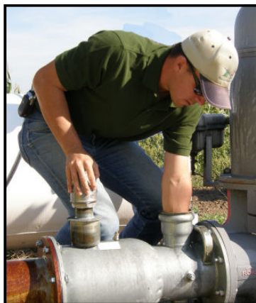
Nolan Little, Tri-Basin NRD Water Resources Technician, conducts a routine chemigation inspection.
